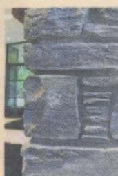
French stonemasons helped craft details like this schist wall.
